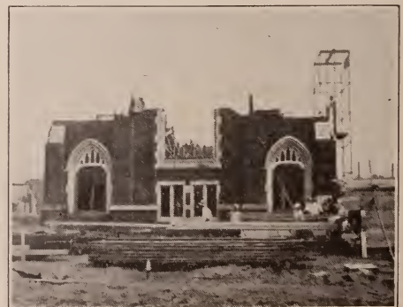
BETHANY CHURCH, CUYAHOGA FALLS, OHIO In Course of Erection
